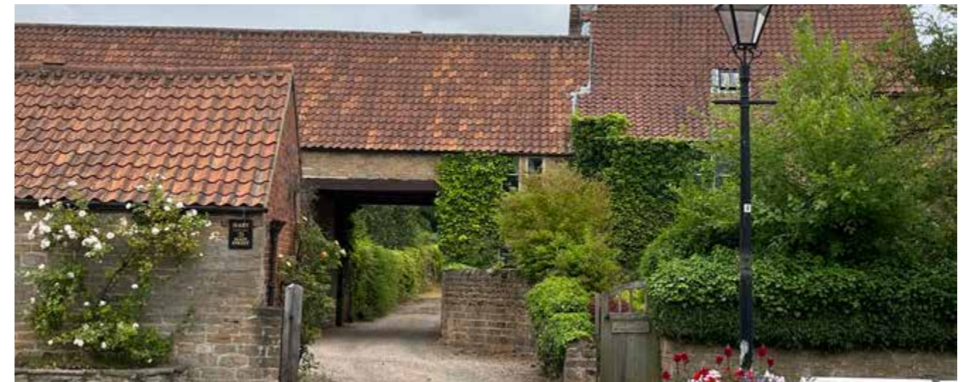
Oversailing roof to farm yard entrance
