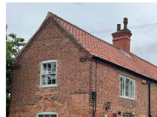
Stepped bricks beneath eaves
