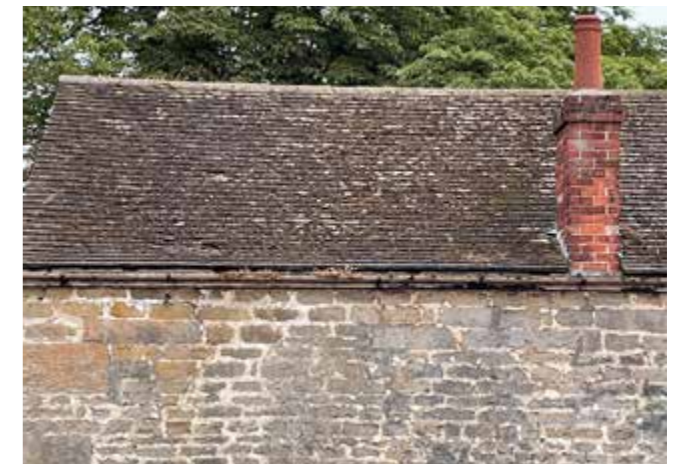
Limestone walls and roofing tiles with red brick
