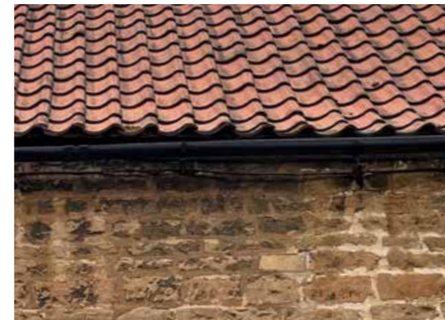
Typical clay pantiles over limestone walls
