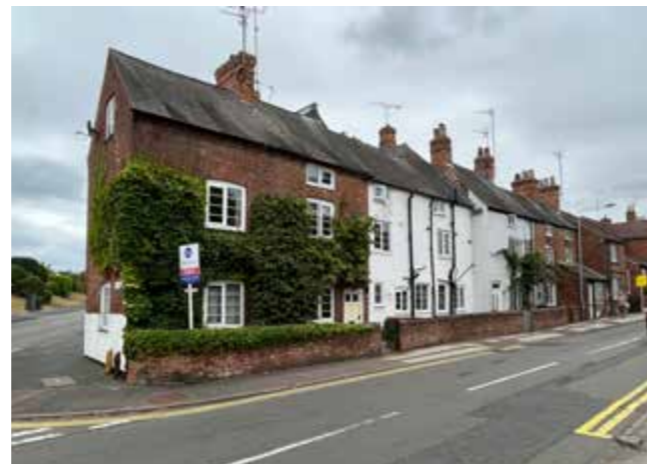
3 storey frameknitter's workshop with windows lining up
