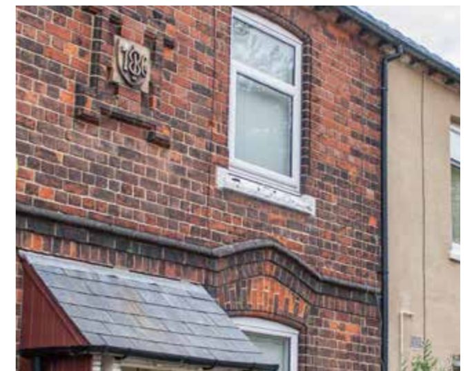
Canopy, corbelling and crest detail
