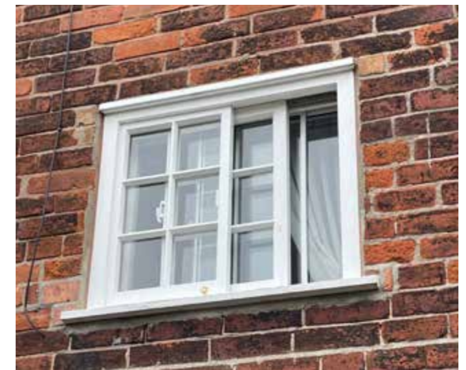
Sliding Yorkshire sash windows are typical
