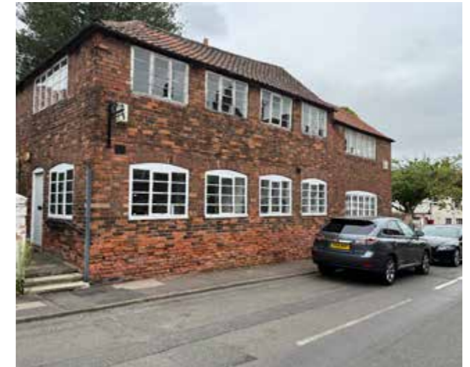
2 storey frameknitters workshop with arched windows
